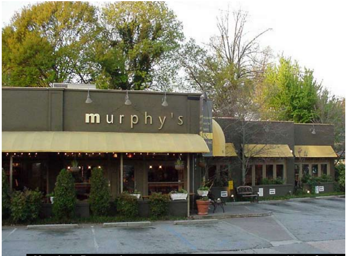
Murphy's Renovation Atlanta, Georgia
